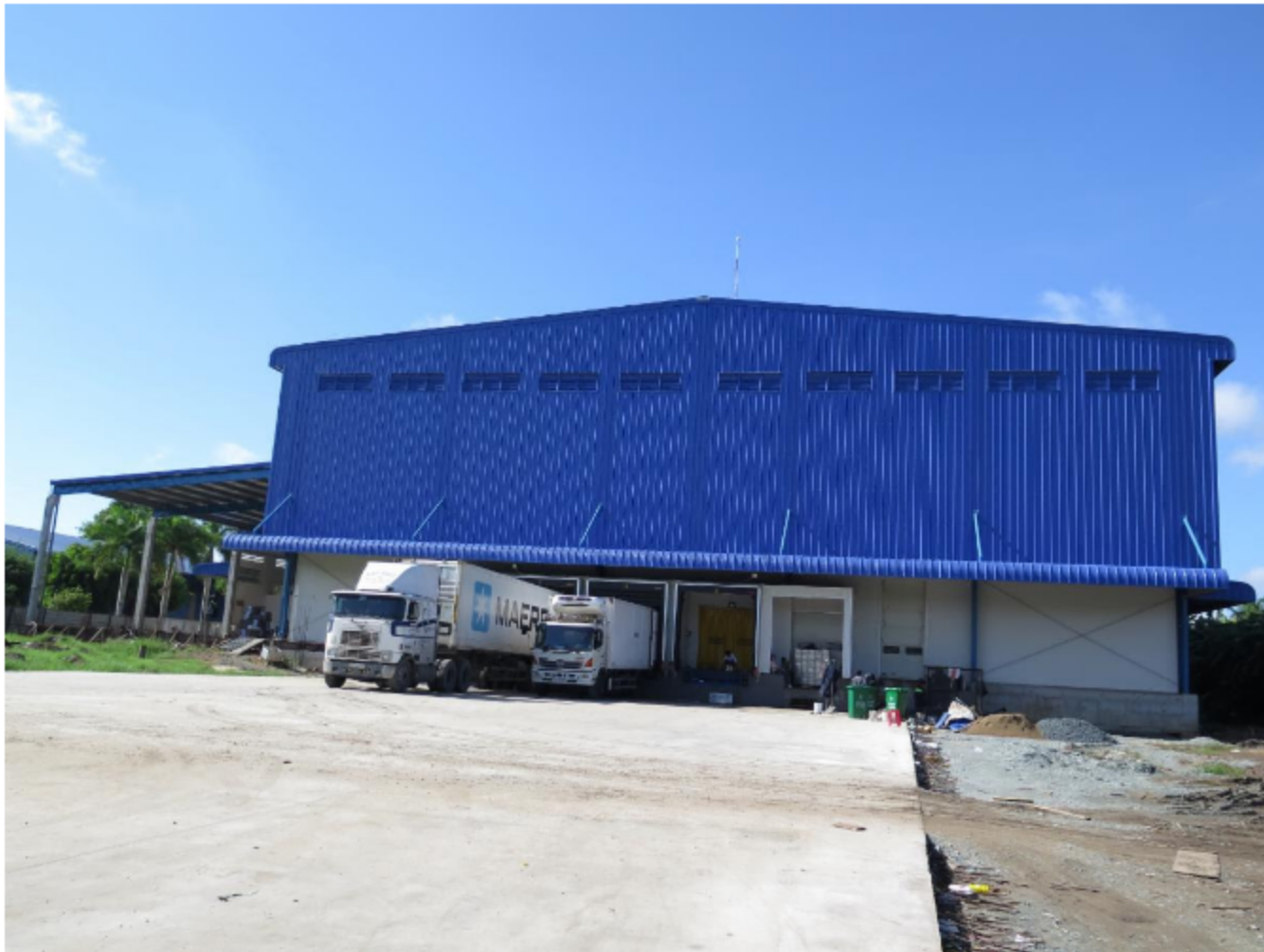
Van Duc Tien Giang's cold storage under construction
