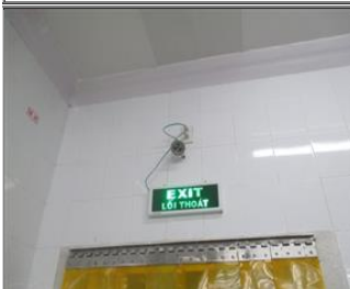
Photo of fire safety equipment C-Emergency exit light and exit sign.JPG
