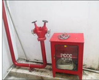
Photo of fire safety equipment C_Fire hose and fire hydrant system.JPG
