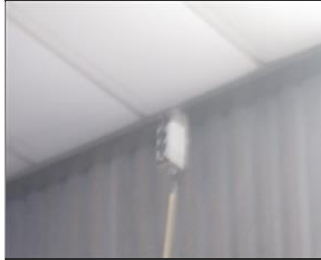
Photo of fire safety equipment C_Beam laser automatic fire alarm system.JPG
