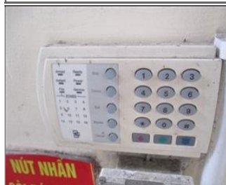
Photo of fire safety equipment C-Fire alarm control panel.JPG
